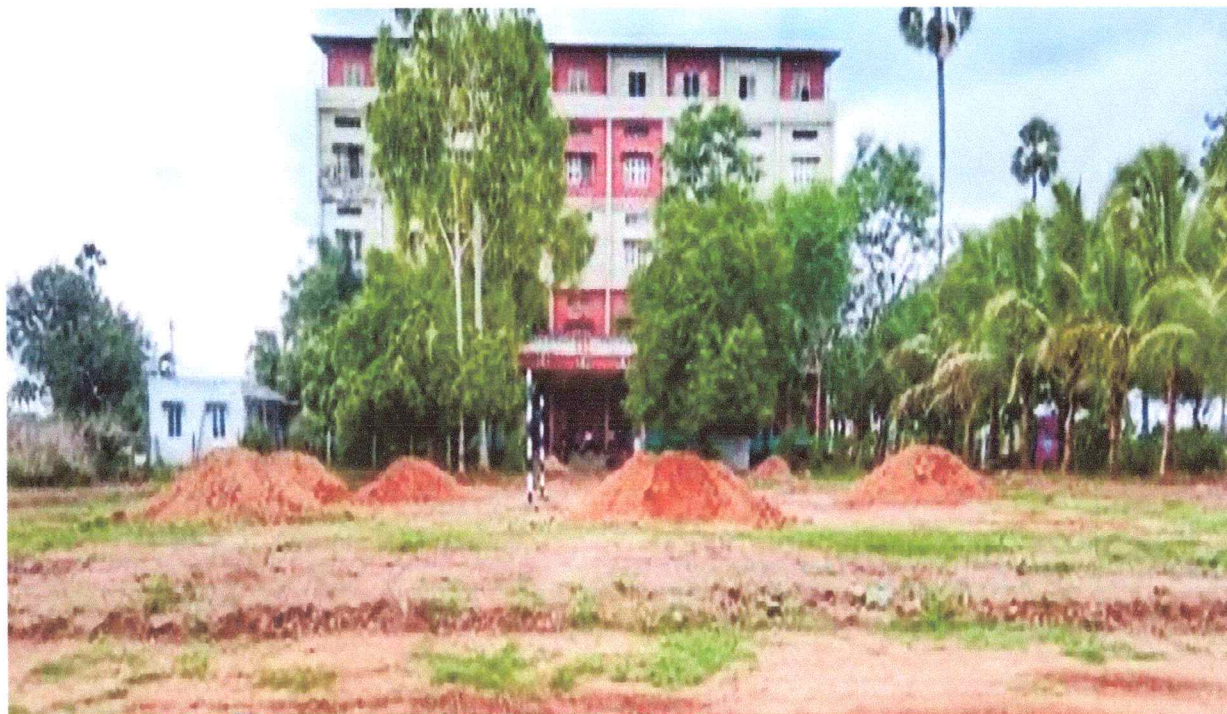
Fig.1: AIPS Campus Building
