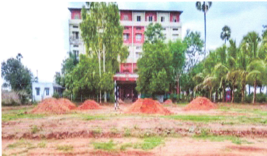
Fig.1: AIPS Campus Building
