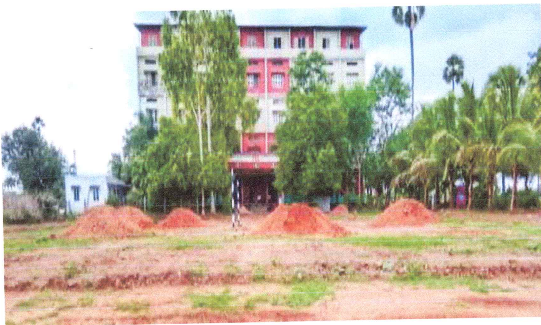
Fig.1: AIPS Campus Building
