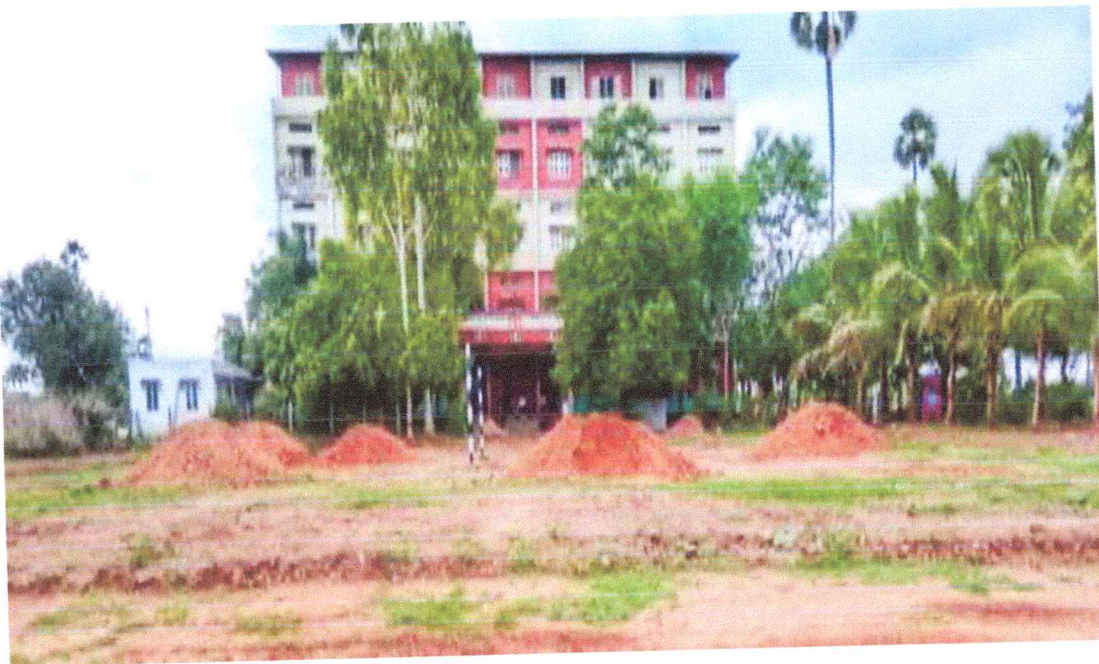
Fig.1: AIPS Campus Building
