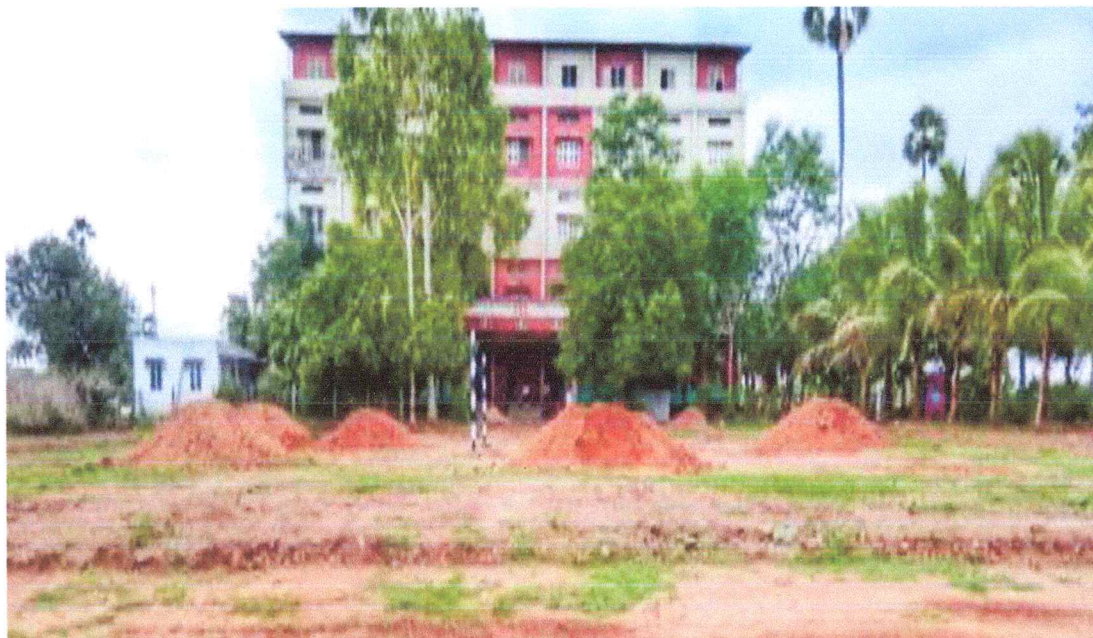
Fig.1: AIPS Campus Building
